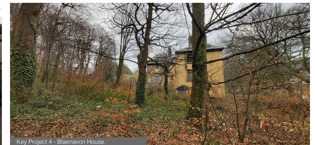
Key Project 4 - Blaenavon House.
