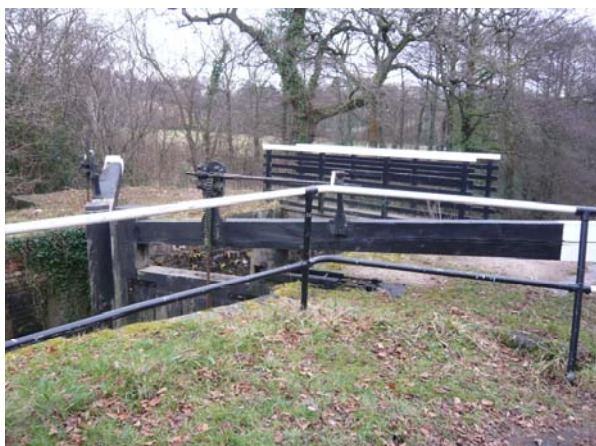
Tamplin Lock gates and footbridge
