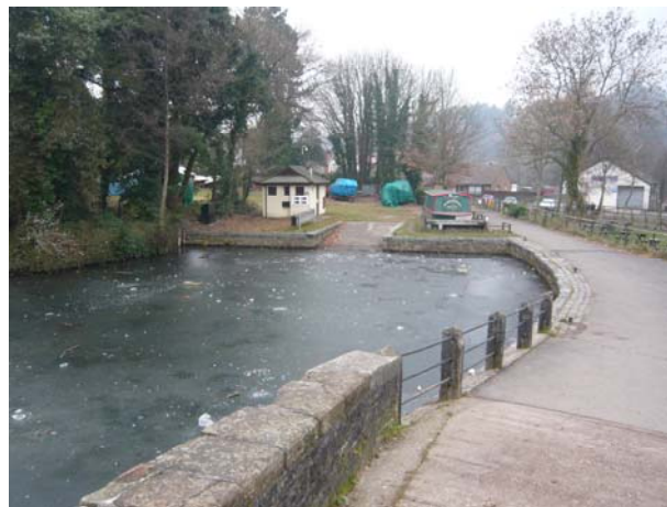
Stone edgings and cobbles at Pontymoile basin
