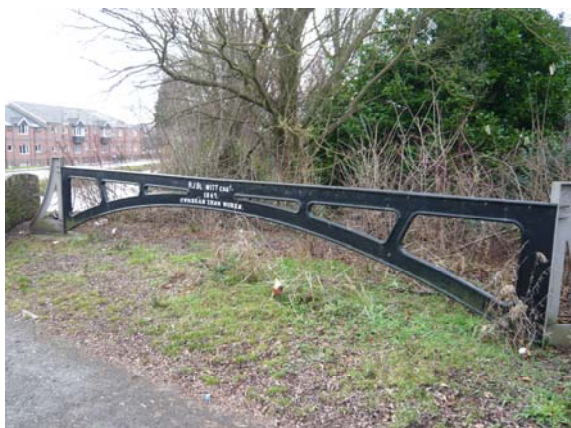
The 'De Witt' bridge girder dated 1847
