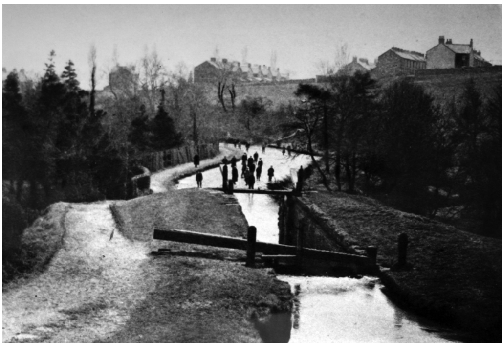
A view southwards looking across the culvert taking the Blaen Bran beneath the Canal at the '5 Locks'
