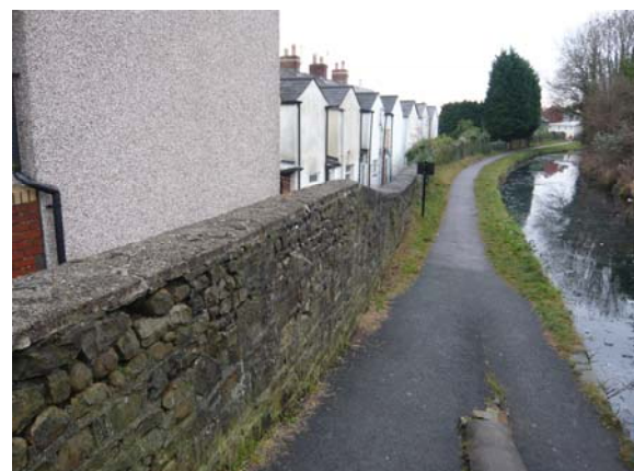
Rear boundary to terrace along Station Road
