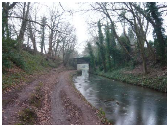
Canal cutting looking towards Pontypool Road Bridge (Bridge No. 53)
