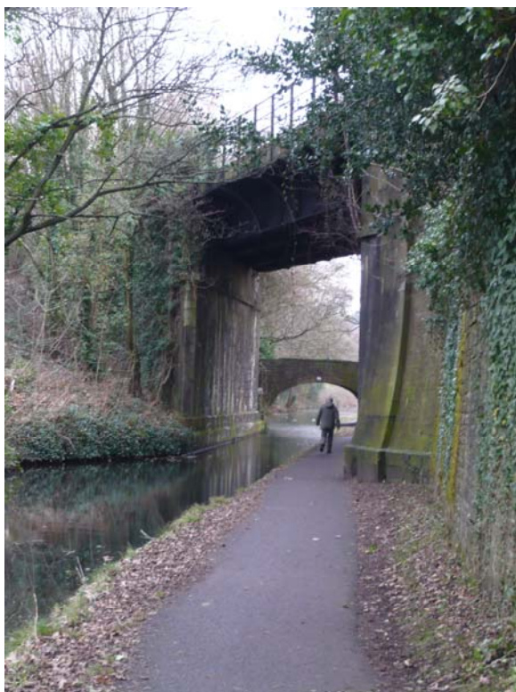
Former Railway Viaduct looking northwards to Coed y Gric Bridge (No. 51)
