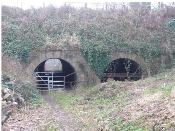
Listed Tram Road Tunnels beneath the Canal
