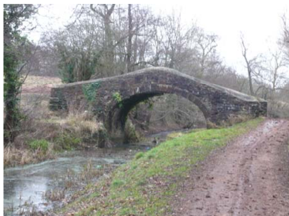
Bridge south of Tamplin Lock
