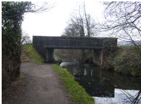
Modern concrete bridge (No.46)
