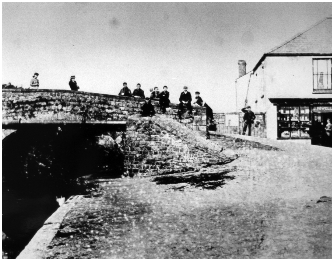
A view of the eastern side of Crown Bridge (Bridge No.48), the shop to the left although much altered still stands as a residence today
