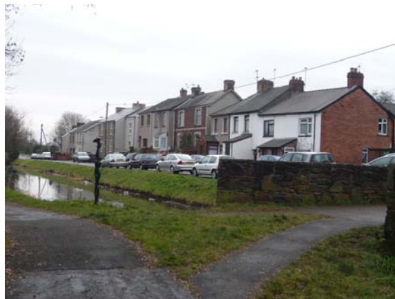
Properties along Ty Coch Road
