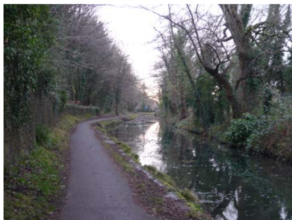
Canal and retaining wall to towpath looking south
