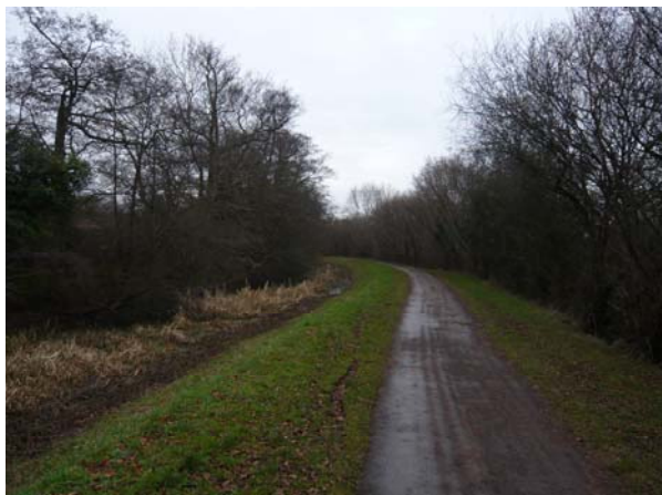
Reed growth in the Canal south of Tamplin Lock
