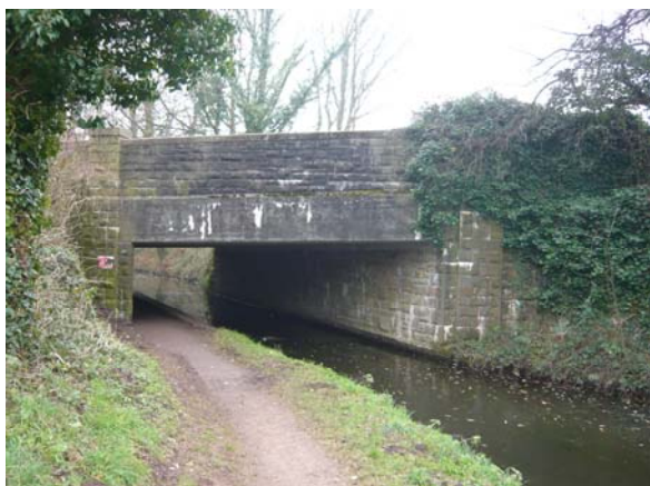
Jockey Bridge (No. 55)
