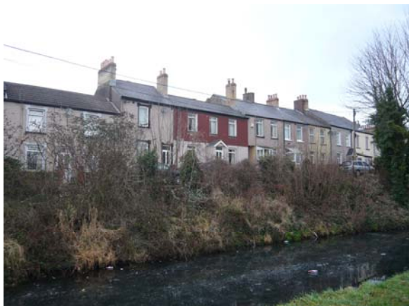
Terraced housing along Bridge Street
