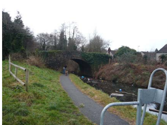
View south to Solomon's Bridge (No.47), including GWR post to west bank
