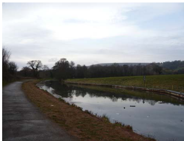
New mooring basin near Sebastopol
