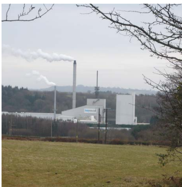
View from atop Bridge No. 46 to the east
