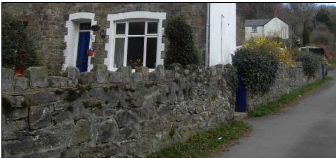
Example of a stone garden wall linking houses with similar materials
