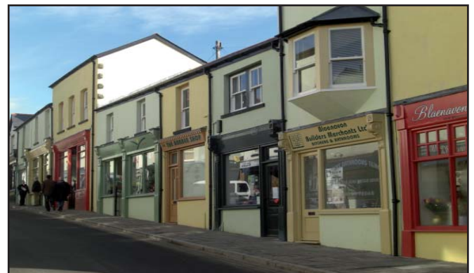
Extensive improvement has taken place within the retail development in Broad Street, giving a significant lift to the character and ambience of the area.
