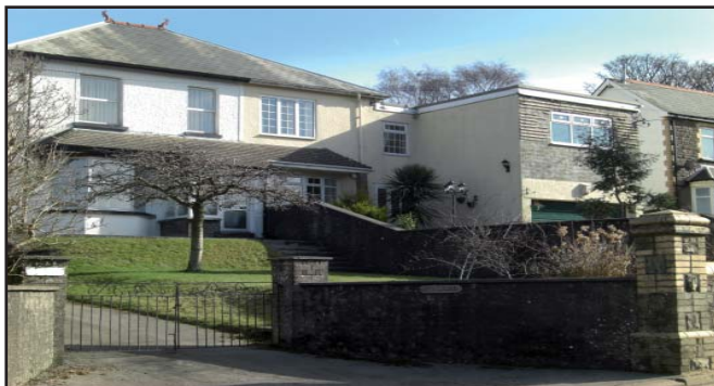
Extensions to buildings need to be sympathetic and responsive to the scale, form and character of the original structure. Usually an extension to the front of the building will break the integrity of the building line. The flat roof and crude elevational treatment is also detrimental to the character of the street scene.
