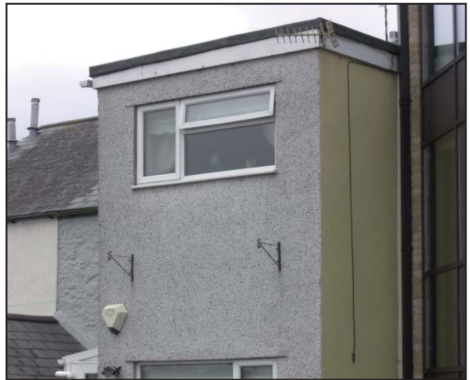
Rear extensions with flat roofs and in materials that do not match the original building do not integrate well with the overall structure giving the appearance of a separate and somewhat alien mass, bolted on to the building.
