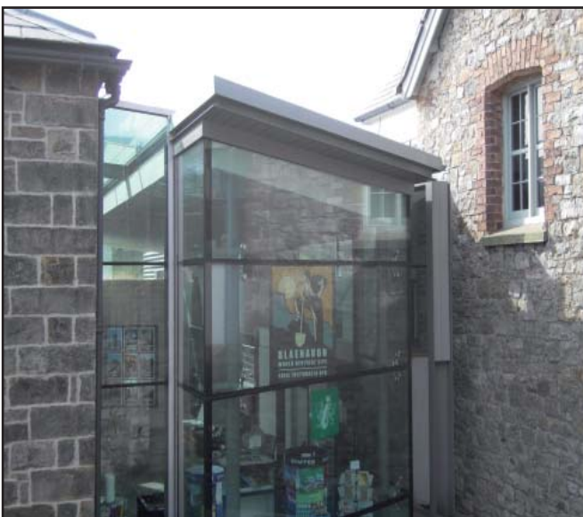
This example of a contemporary design approach to an extension to a heritage building demonstrates careful selection of materials to complement the original building. If the design is clearly of a different era, it is usually better if there is a very clear visual separation between old and new. A glazed structure allows the original, more massive stone building, to retain its clarity of form. Keeping the height of the new building below the eaves line allows a neater junction between the different elements.
