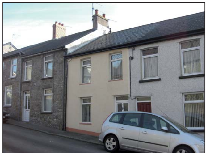
Render should be avoided on stone buildings and should be removed if possible. Where a rendered finish is used it should be smooth (centre) rather than textured (right).
