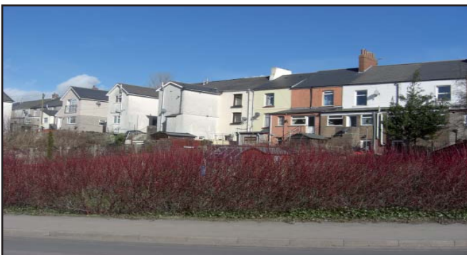
Perimeter block development can help to prevent exposed rear elevations being visible from public areas, as illustrated here.
