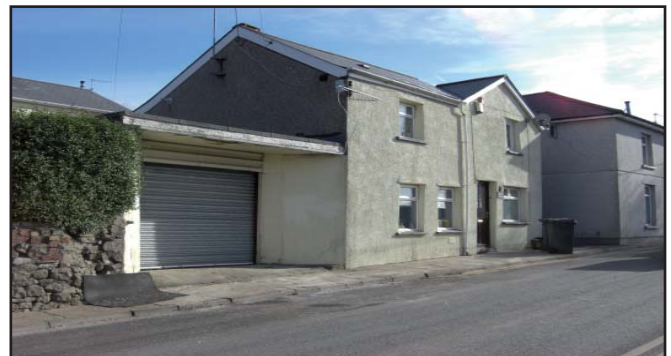
Extensions to buildings need to integrate with the form of the original building. The roof is a particularly important part of the overall massing of a structure. Flat roofs rarely sit comfortably alongside a setting where pitched roofs are the established form.
