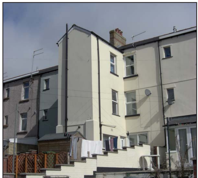
Care must be taken to avoid any extension from being over-dominant in the overall massing of the building, or terrace as a whole. In this example, a two storey extension, rather than three, would have allowed the roof line of the new part to be below the height of the original and be subservient and far less visually obtrusive.
