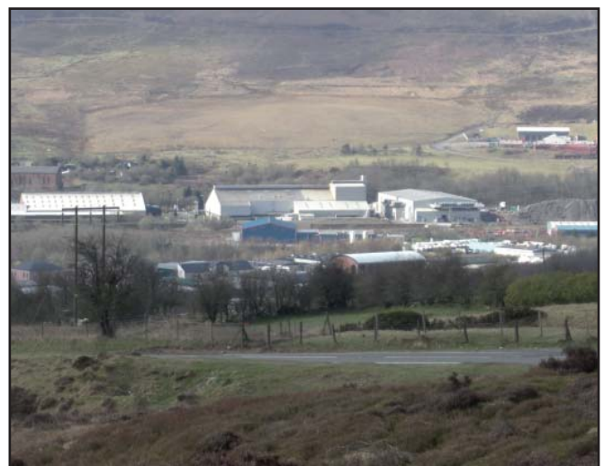
In distant views, from higher ground, it is the roof which is the most prominent element of the building. The colour and reflective qualities should be considered carefully to minimise the visual impact on the landscape setting of the area as a whole.
