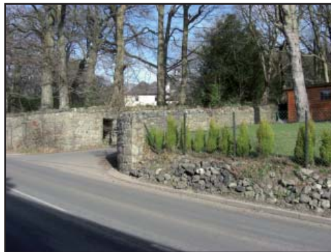
Stone boundary walls form an important component in the streetscape of the area and should always be retained. Hedges and timber fences do not provide the same character and qualities, particular to the WHS area.
