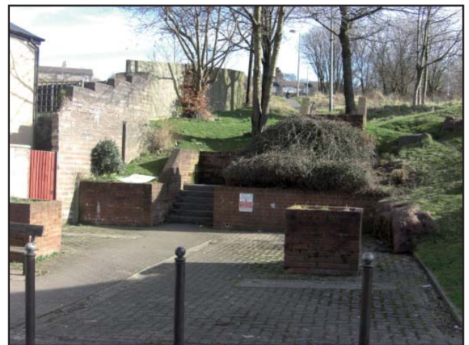
The topography of the area necessitates steps which should be retained in their original stone material (above top). Poor designs and the inappropriate use of brick should be avoided (above and middle).
