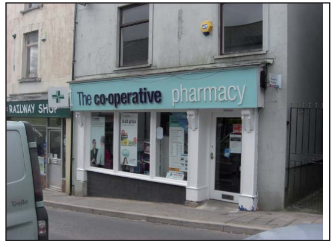
The fascia should not be too large, as in this example in Broad Street, to avoid an imbalance of proportions and over-dominance of the elevation as a whole.
