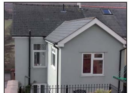
Rear extensions with pitched roofs and in materials that match the main structure are much better integrated than those with flat roofs.
