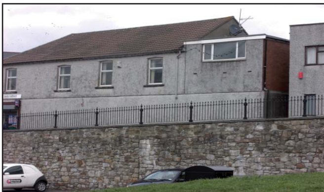
Whether for a 19th century heritage building or a later development as shown here, the fundamental principles of a design for a new building, or an extension to an existing one, should be to respond to the prevailing context of the area. Flat roofed structures with inappropriate windows, proportions and design, crudely 'bolted onto' the existing building is a poor response and damages the street scene as a whole.
