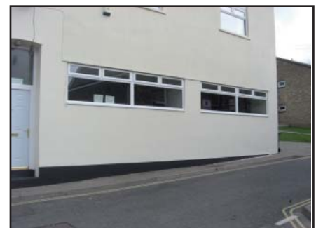
The vertical emphasis of the windows openings is an important part of the character of the area. Horizontal designs look completely out of place and should be avoided.
