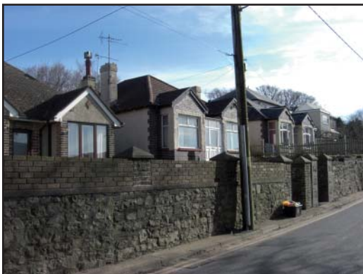
Boundary walls are a very important feature throughout the WHS area and make a very significant contribution to the character of the area. Where stone walls are provided they should not be repaired or extended with any other material.
