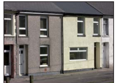
The combination of changes to the window openings and the window materials and design has a major cumulative effect in diluting the qualities of this terrace.
