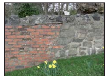
Stone walls should be retained where possible. The use of brick is alien to the overall palette of materials of the heritage of the area and should be avoided.
