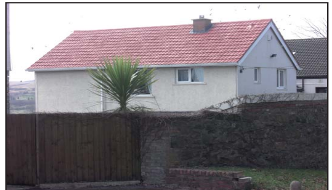
Brightly coloured tiles are particularly alien to the palette of materials and natural tones of the landscape and traditional buildings in the WHS, are unacceptable and should be avoided.
