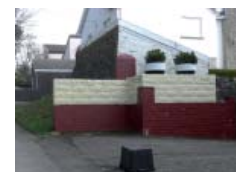
Painted or unpainted blockwork and brick walls should not be used.
