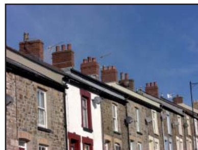
The regular rhythm of the chimneys forms an important and dominant element in the streetscape, emphasised by the simplicity of the overall form and detailing of the terraced buildings.
