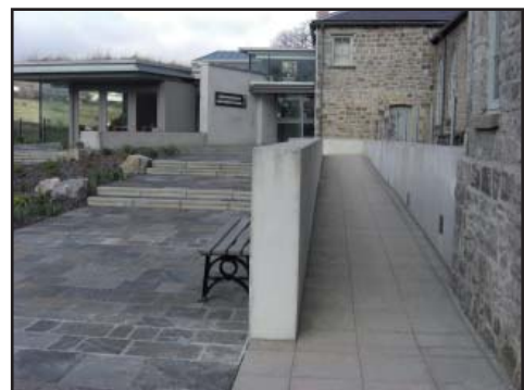
Where ramps are provided for disabled access they should be considered as part of the design as a whole and fully integrated, as successfully shown in this example.
