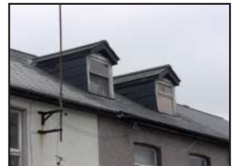
The proportions of the windows and window frames within the dormers needs to be carefully considered and should match the overall 'rules' that are applied to window openings generally.
