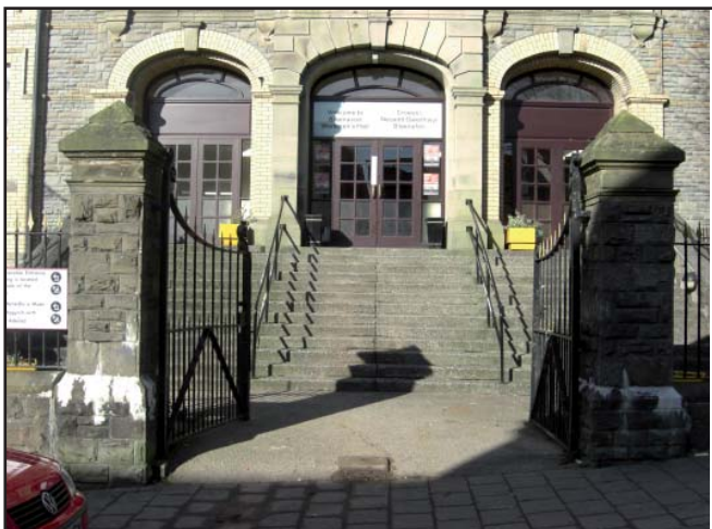
Entrances are an important feature of many of the larger public buildings in the area.
