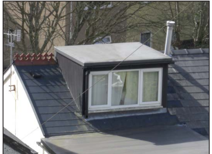
New dormer windows should never project above the roof line, and should normally have a pitched roof and windows in proportion with those in the building as a whole.
