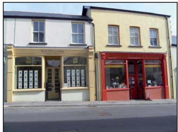
Many of the shop fronts in Broad Street have been reinstated with an attractive balance of variety and consistency, based on historic photos.
