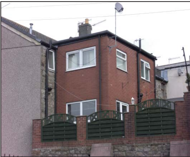
Rear extensions with flat roofs and in materials that do not match the original building do not integrate well with the overall structure giving the appearance of a separate and somewhat alien mass, bolted on to the building.
