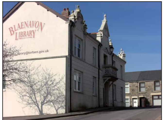
The decorative gable features of the Blaenavon Public Library give it the air and character of a public building.
