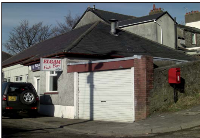
Selection of materials is very important in any extension to an existing building. Matching in and / or being sympathetic with adjacent areas will help ensure a subtle transition and integration of new and old parts of the building.
