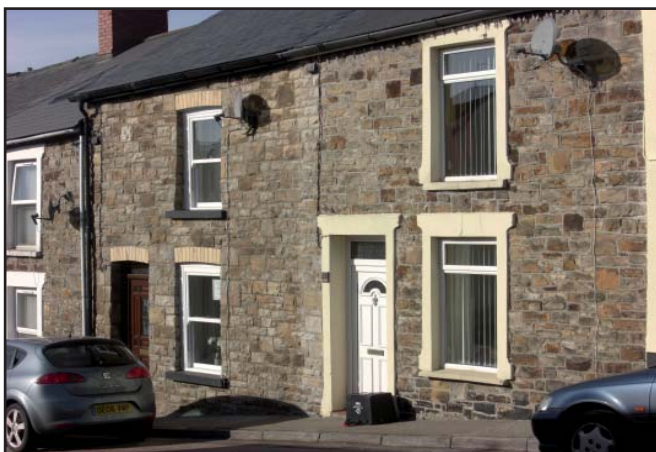
The terraced development of the mid 19th century growth of the town is simple in its basic form, which gives additional importance to the details of windows and doors and the small architectural details of the building. In these examples, although the window openings have been retained in their original sizes, some of the proportions of the window designs are not in their traditional proportions.
