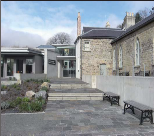
There are few examples of contemporary design in the area, and none for residential buildings. It can be successful when the standard of design and materials is maintained. When integrated with heritage structures, a clear distinction between new and old is necessary, as shown here.
