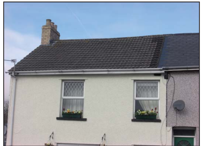
Where re-roofing is necessary it should always be in slate. Tiles are not only less in keeping with the area but can also cause structural problems as they are often heavier than the original material and can cause problems with the structural timber frame within the roof.
