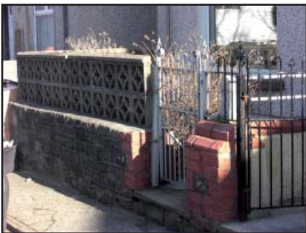
Stone walls should be retained and any repairs carried out in the same material. Mixing stone, brick and other concrete blocks is not appropriate.
