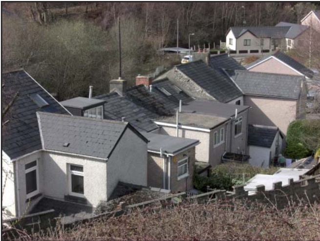
The pitched roofed extensions form a more unified and integrated overall structure than the flat roofed examples.
