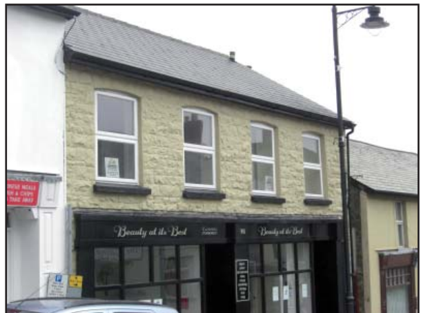
Natural stone should not be painted under any circumstances. It can lead to the disintegration of the stone and is likely to cause greater problems and costs in the long term.
