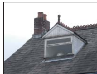
The proportions of the windows and window frames within the dormers needs to be carefully considered and should match the overall 'rules' that are applied to window openings generally.
