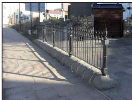
A rounded stone coping to a wall, or in this case as an upstand in itself, supporting railings, is a feature in the public spaces of Blaenavon providing a boundary treatment that integrates very well with the paving, boundary walls and stone buildings around it.
