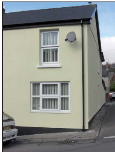
Designs in Upvc, which try to imitate traditional timber sash windows, often look inappropriate, as they fail to match the size and proportions of the elements of original designs or allow the plane of each component to be replicated. They often have a tilting opening mechanism that makes them appear even more incongruous when they are open.
