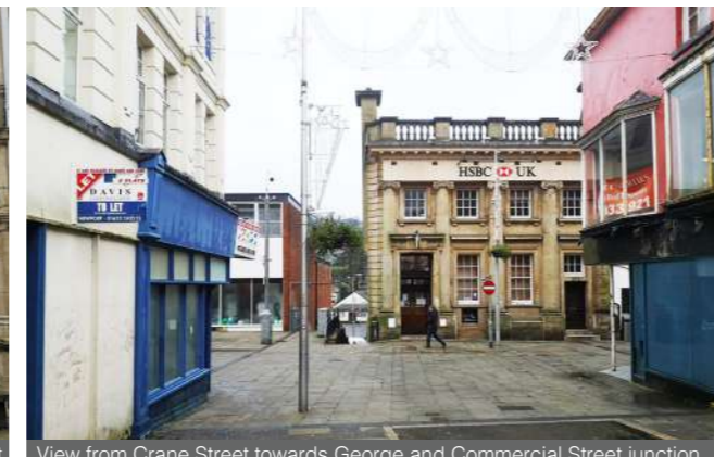
View from Crane Street towards George and Commercial Street junction.
