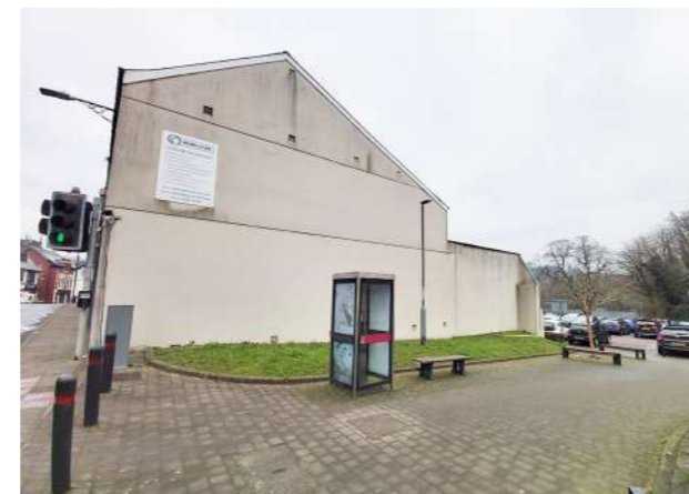
Pedestrian link from Clarence Street to the surface car park.
