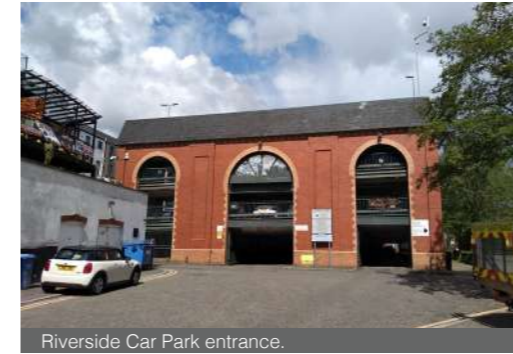
Riverside Car Park entrance.
