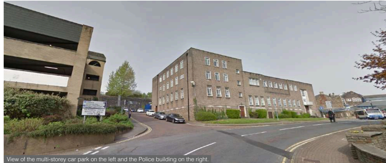
View of the multi-storey car park on the left and the Police building on the right.
