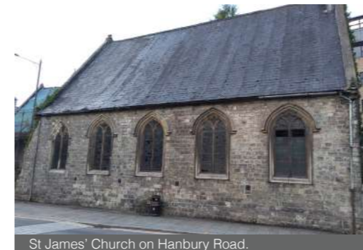
St James' Church on Hanbury Road.
