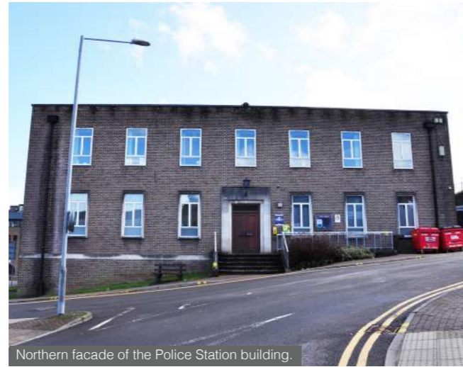
Northern facade of the Police Station building.
