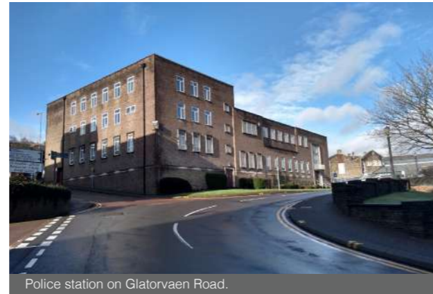
Police station on Glatorvaen Road.
