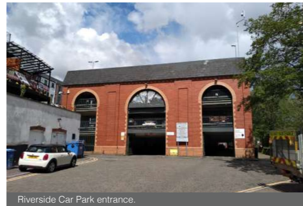
Riverside Car Park entrance.
