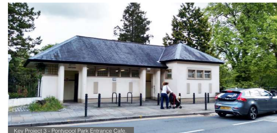
Key Project 3 - Pontypool Park Entrance Cafe.
