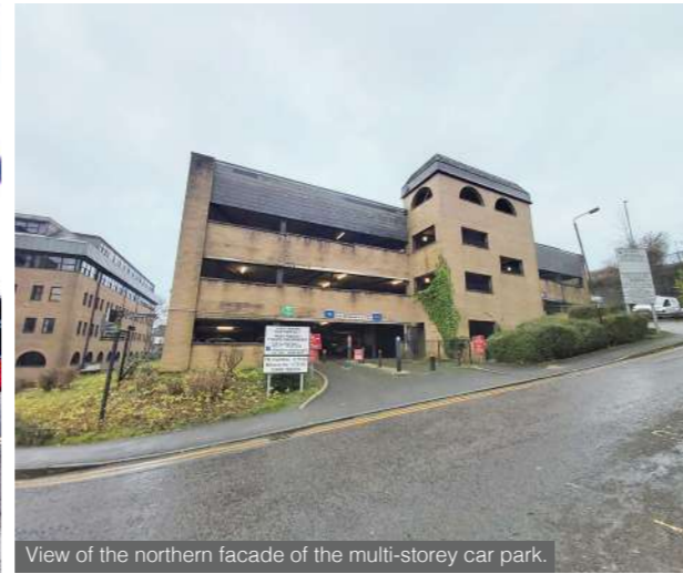
View of the northern facade of the multi-storey car park.
