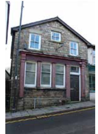
NO 15, BROAD STREET (W SIDE)
