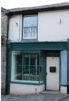
NO 16, BROAD STREET (W SIDE)
