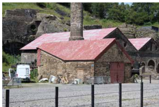
Buildings within Blaenavon Ironworks
