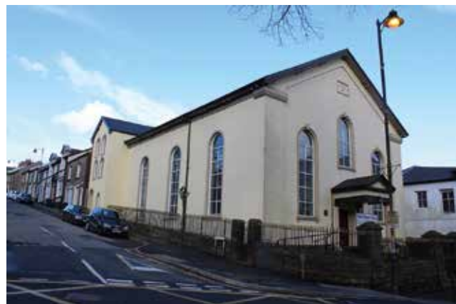
HOREB BAPTIST CHURCH, CHURCH ROAD (NE SIDE)
