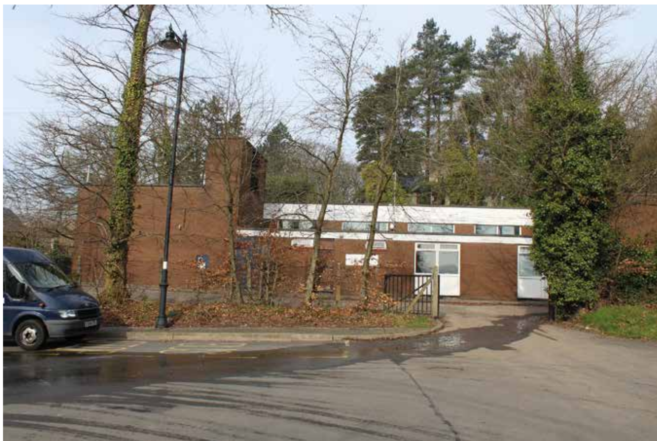
Telephone Exchange work shop
