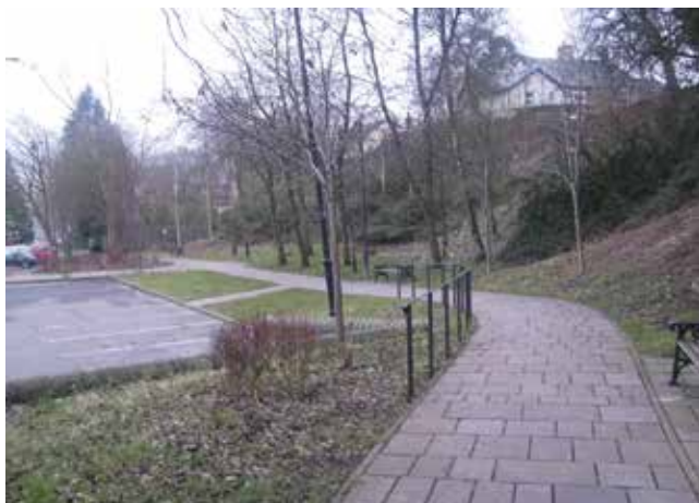
On the boundary of the Broad Street Car Park and Waun Villa
