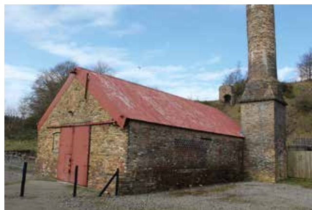
STORAGE SHED AND ATTACHED CHIMNEY, BLAENAVON IRONWORKS
