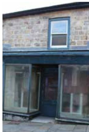
NO 17, BROAD STREET (W SIDE)
