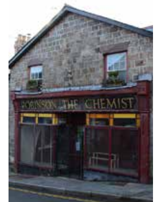
NO 19, BROAD STREET (W SIDE)
