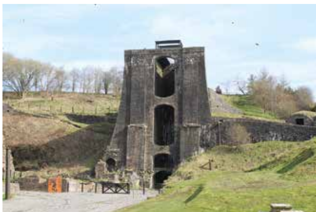
BALANCE TOWER, BLAENAVON IRONWORKS
