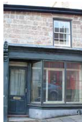
NO 18, BROAD STREET (W SIDE)
