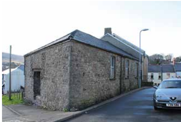
FORMER SCHOOL-ROOM TO REAR, BROAD STREET (E SIDE)
