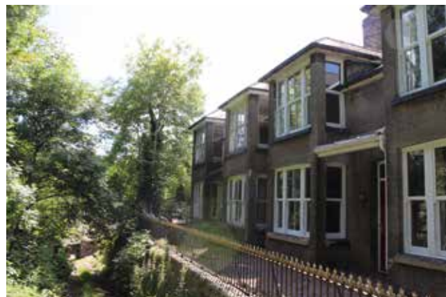
FORMER BLAENAVON SUBSCRIPTION HOSPITAL
