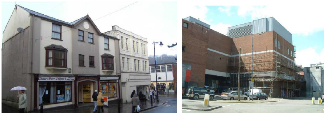
Examples of unsuccessful new designs – a pastiche approach with inaccurate proportions and details and a contemporary building which disregards scale, elevational treatment & materials while facing the entrance to the Conservation Area.
