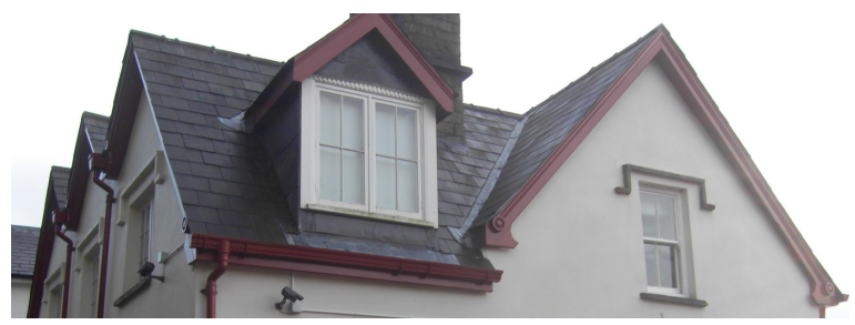
Dormers can provide variety and interest to the roofline and the opportunity for attic rooms where the roof pitch is steep enough.
