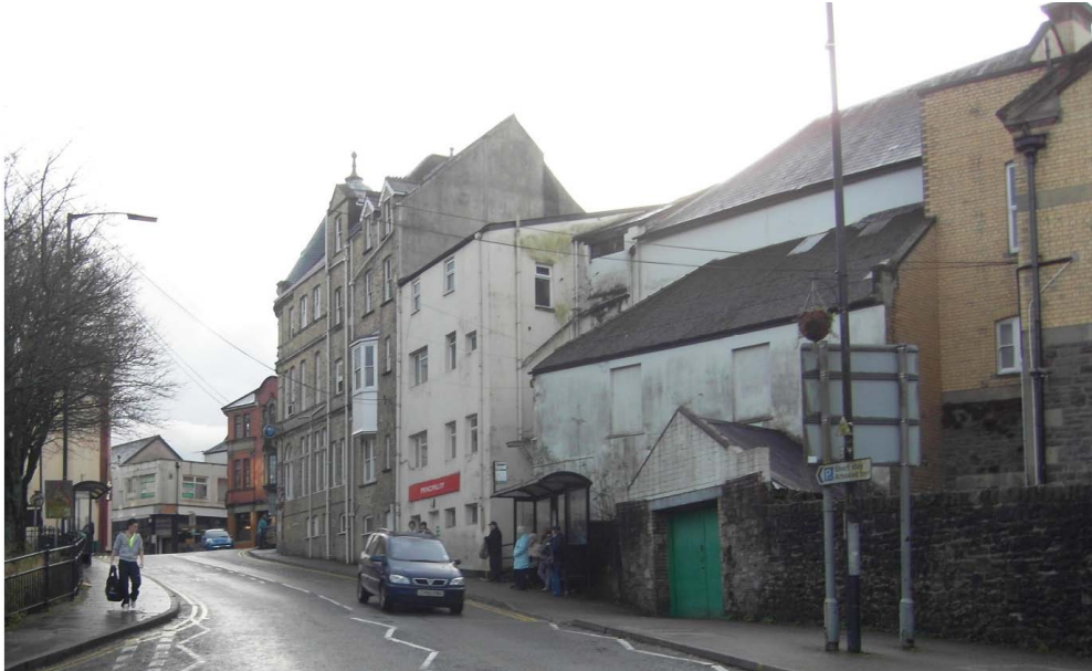
Buildings in a poor state of repair have a detrimental impact on the wider area. This example shows the northern entrance to the Conservation Area looking up Park Road towards buildings on Commercial Street.
