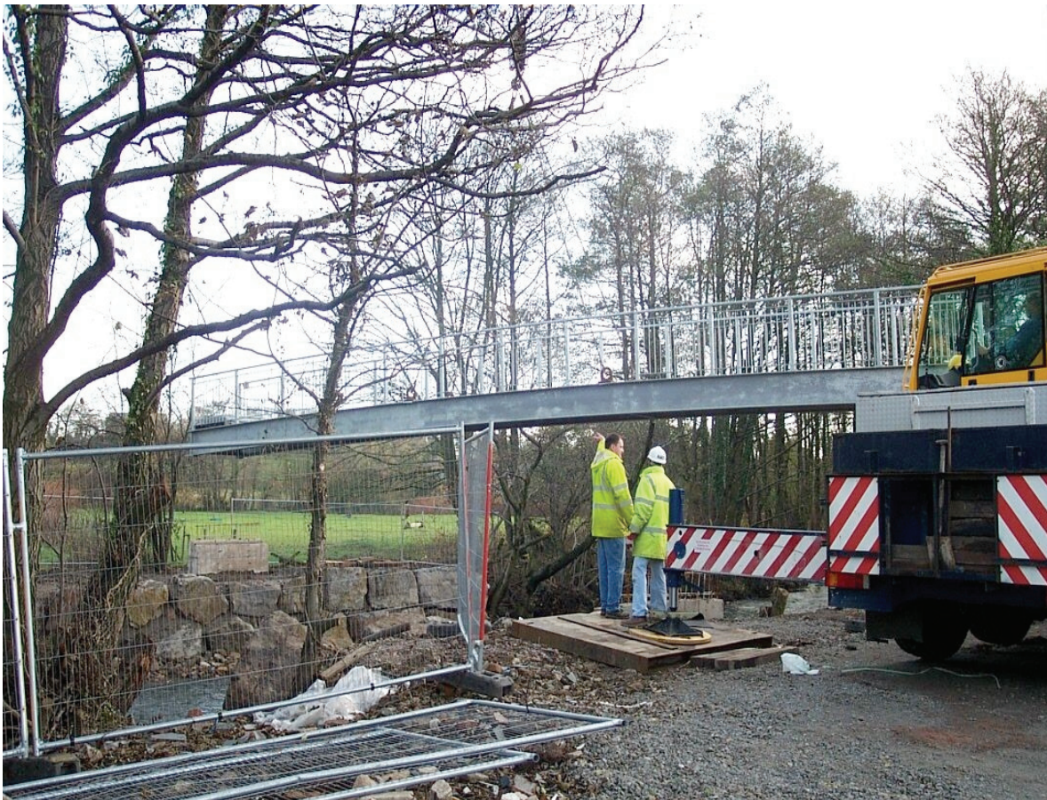
Replacing a footbridge at Pontyfelin at a cost of £65,000
