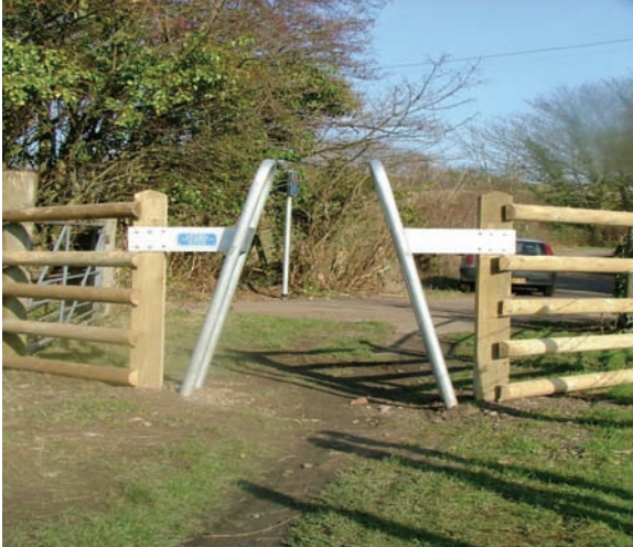
One of the designs of motorcycle barrier used on rights of way
