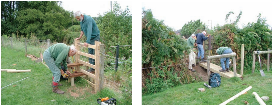
Volunteers helping the Countryside Warden to install a stile and a foot-bridge
