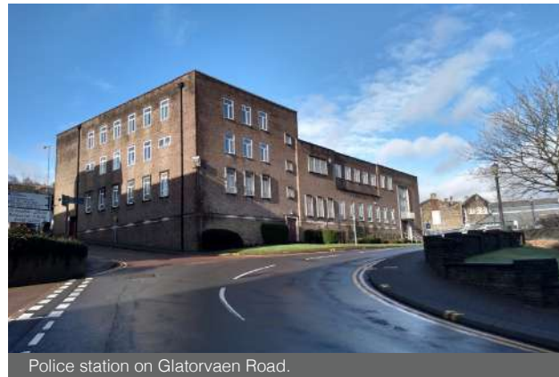
Police station on Glatorvaen Road.
