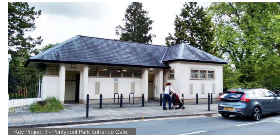
Key Project 3 - Pontypool Park Entrance Cafe.
