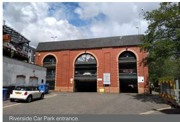
Riverside Car Park entrance.
