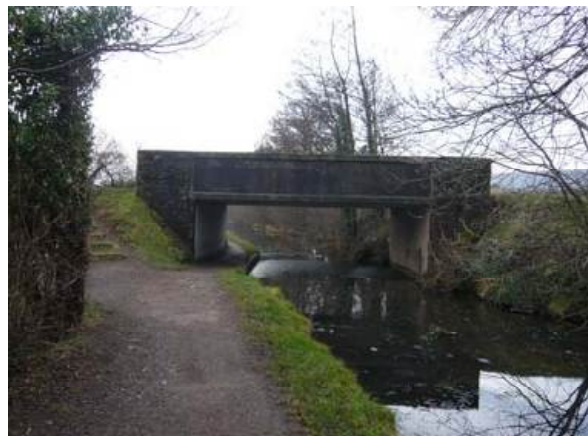
Modern concrete bridge (No.46)
