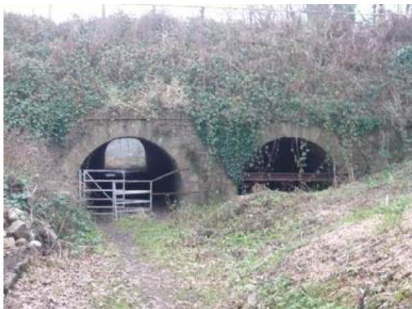
Listed Tram Road Tunnels beneath the Canal
