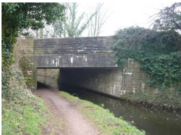
Jockey Bridge (No. 55)
