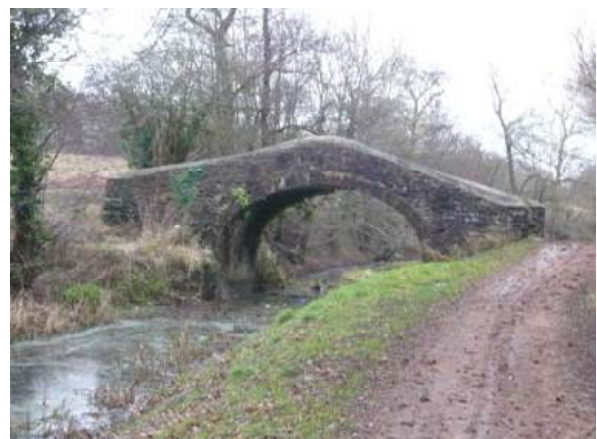
Bridge south of Tamplin Lock
