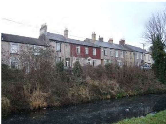
Terraced housing along Bridge Street
