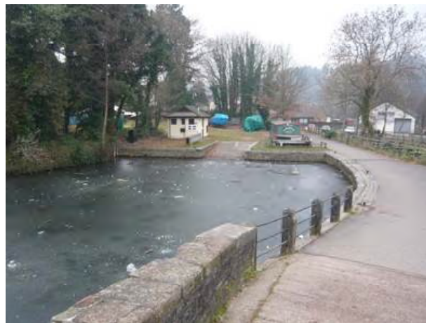
Stone edgings and cobbles at Pontymoile basin
