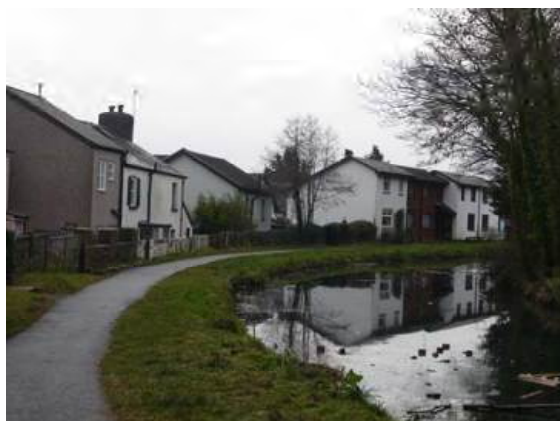
Properties adjoining the Canal along Wern Road
